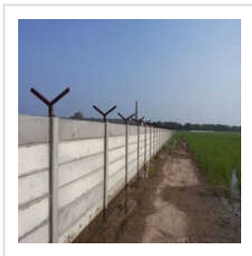
Industrial Boundary Wall
