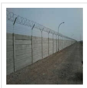
Precast Pre Stressed Boundary Wall
