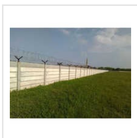
RCC Folding Compound Walls
