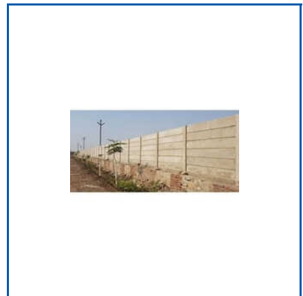
READYMADE PRECAST BOUNDARY WALL
