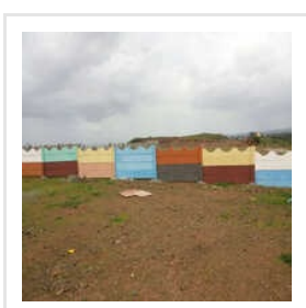
RCC Residential Compound Wall
